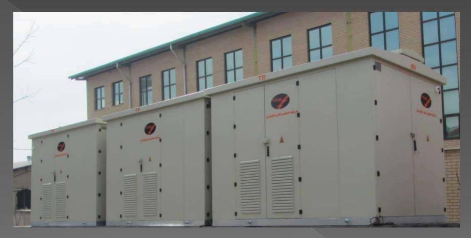
The compact substation is asset of transformers, low voltage switchgear and medium voltage switchgear
