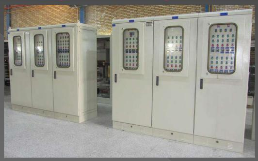
Protection against water pressure at the pressure of 100 KPA And protection against objects larger that 1 millimeter
